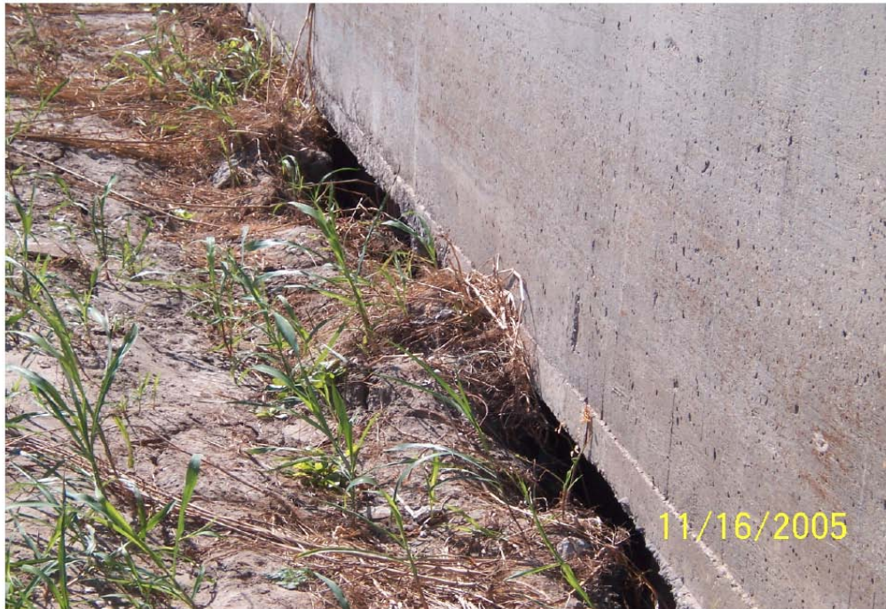
Figure C-1. Gap on the canal side of the Michoud Canal I-wall in New Orleans after Hurricane Katrina
